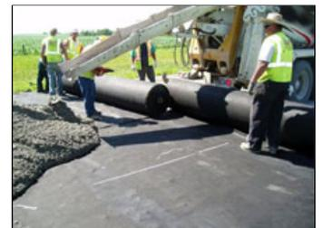
Geotextile bond breaker between paver and ready-mix trucks
