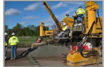
The third test section (cell 70) was constructed of a PG64-34 Superpave hot-mix asphalt (HMA) overlay surface placed over a recycled concrete mix. The HMA pavement will incorporate saw and seal over the transverse PCC joints to control reflective cracking from the underlying recycled concrete mixture.
