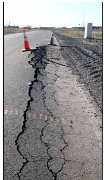
MnROAD farm road test track damage
