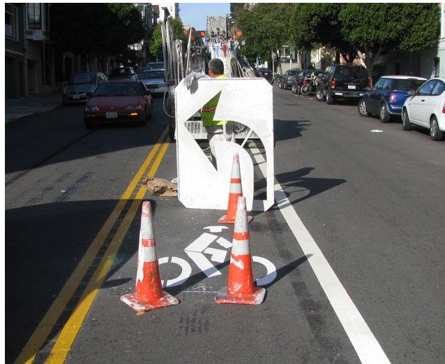
Figure 1.3: Road Marker Painting using Stencils [6]
