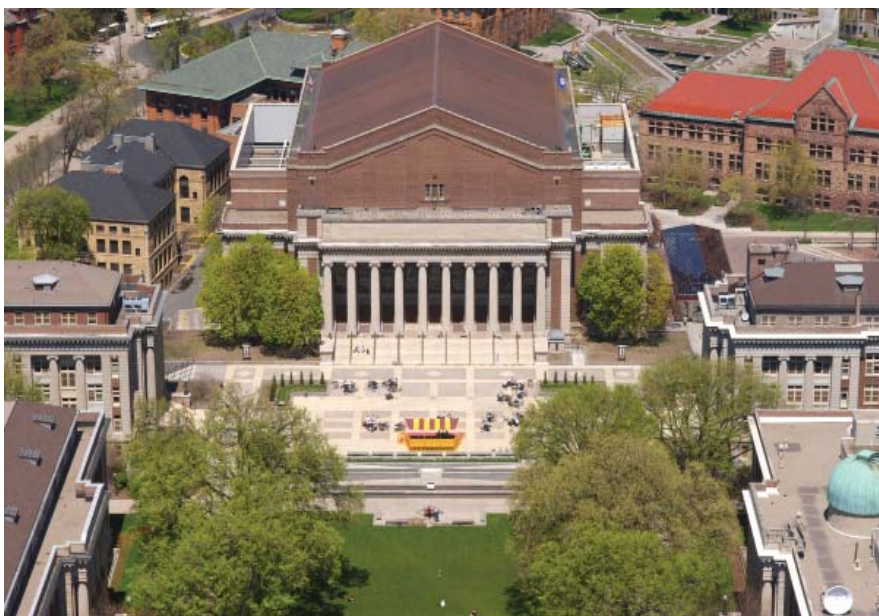
Northrop Auditorium reopened in April 2014 after renovation work. OGC developed form agreements for the use of the renovated space.
