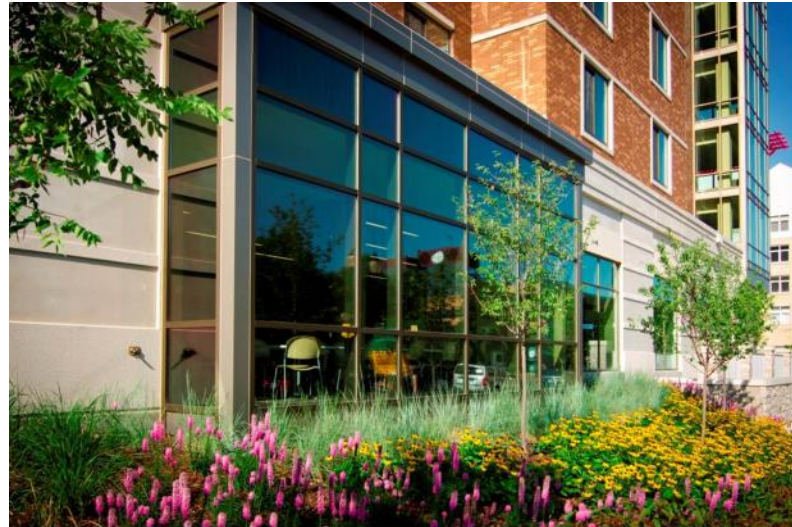
: Residence Hall, UMMC Photographer: Joe Brennan
