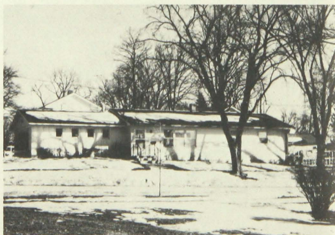
Figure 17. Residual snow pattern on a cold-roof house specifically designed for ice-dam immunity.
