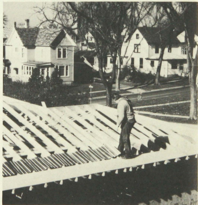
Figure 24. Workman applying air passage protector along eaves.
