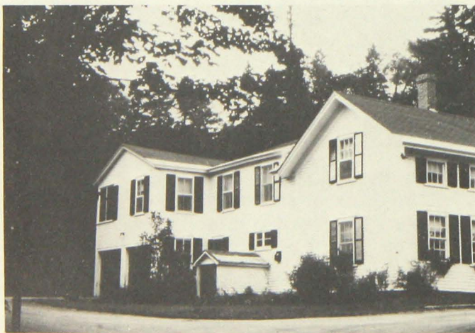
Figure 9. Eave flashings of aluminum.
