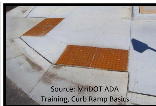
Figure 4.9 Detectable Warning Surfaces (Truncated Domes)
