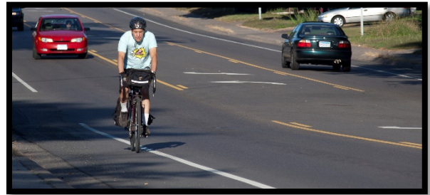
Figure 7.15 Pavement Striping/Road Diet
