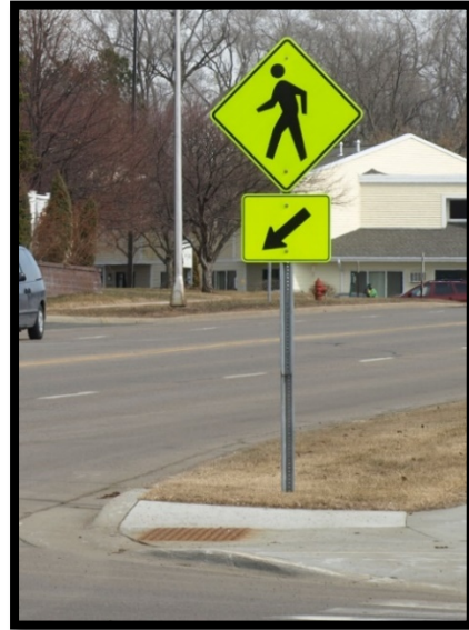
Figure 7.5 Pedestrian Crossing Warning Sign with Down Arrow
