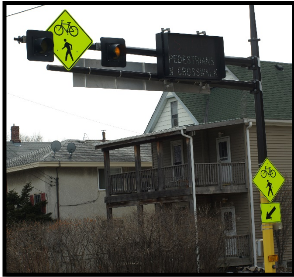
Figure 7.10 Overhead Flashing Signal Beacons
