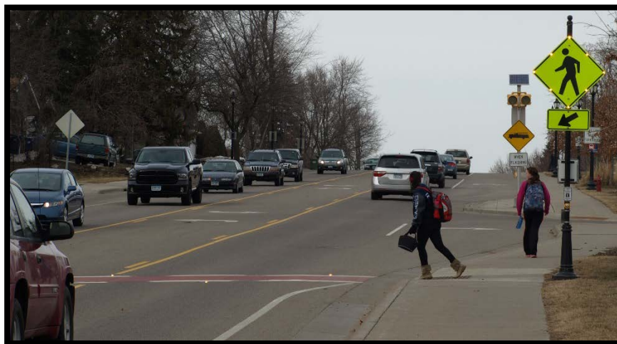
Figure 7.12 In-Road Warning Lights with Edge Lit Warning Sign
