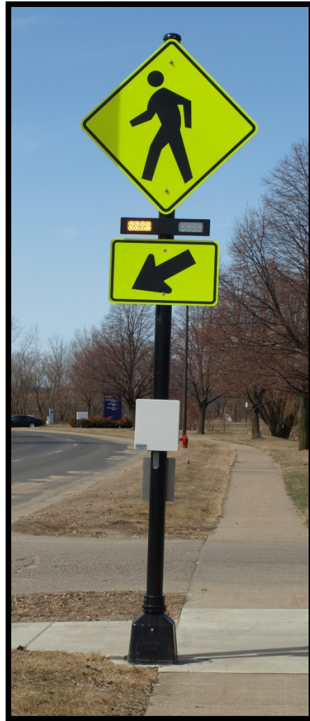
Figure 7.11 Rapid Rectangular Flashing Beacons (RRFB)
