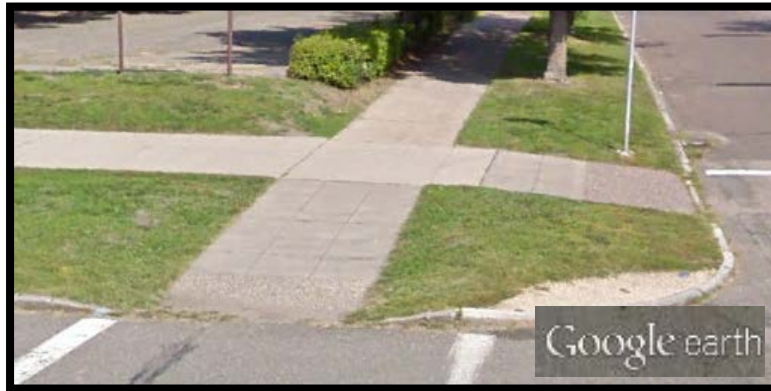
Figure 4.10 Curb Ramps with Landing and No Truncated Domes [14]
