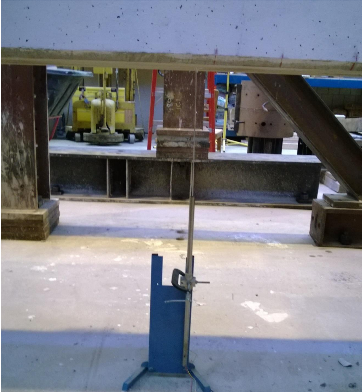
Figure 3-30: LVDT attached at the centerline of the 36M prestressed girder at the displacement controlled actuator location representing the typical placement for the 3 in. LVDT.
