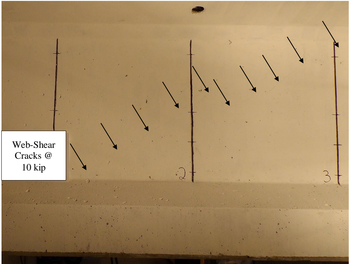
Figure 3-56: Initial web-shear cracks in 45M_24W unloaded to 10 kips applied.
