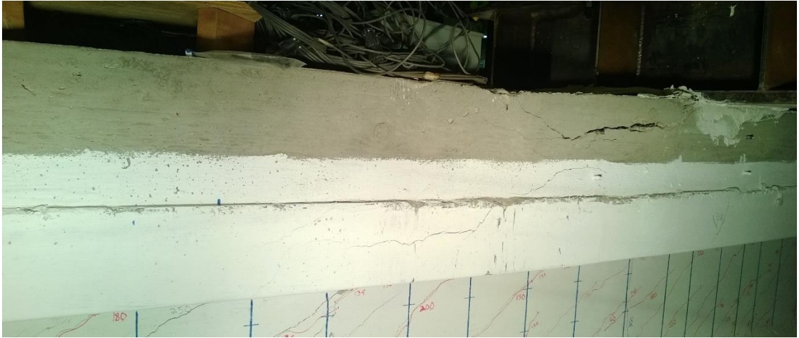
Figure C-38: Deck crushing observed during 36M_8W test.
