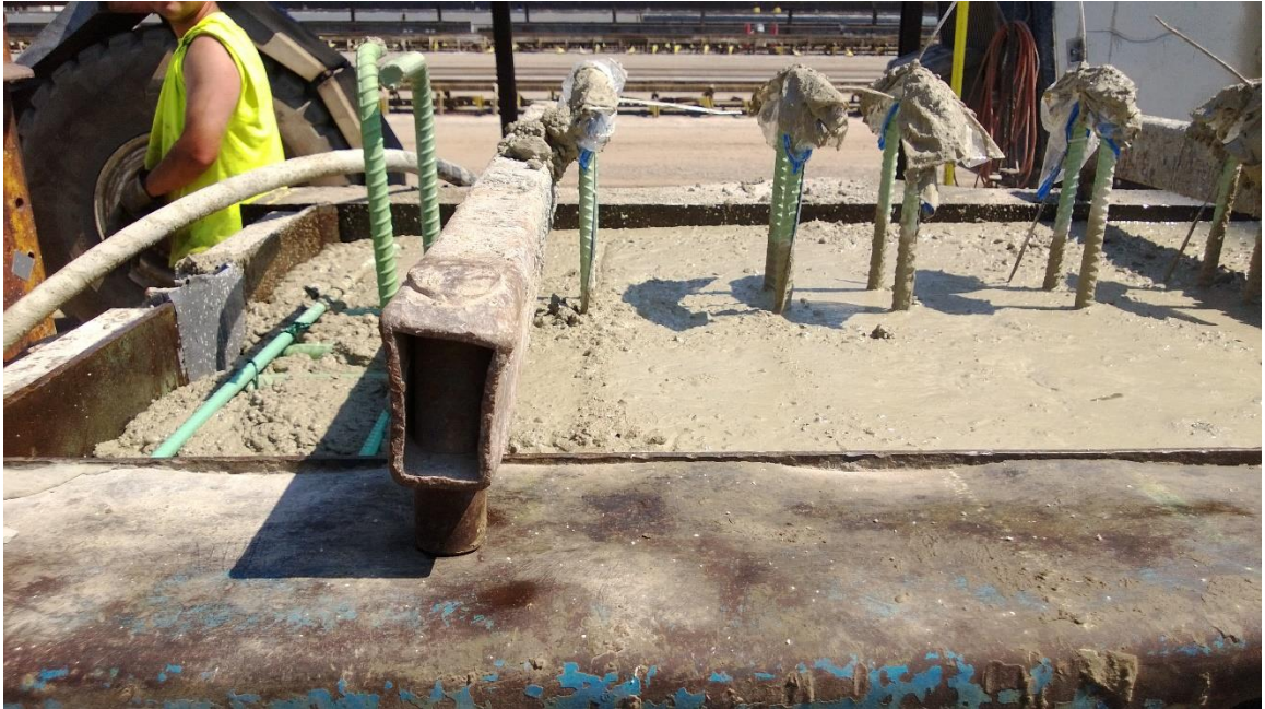
Figure 3-18: Remaining volume in 36M_18F girder end which was filled by a fifth batch of concrete.
