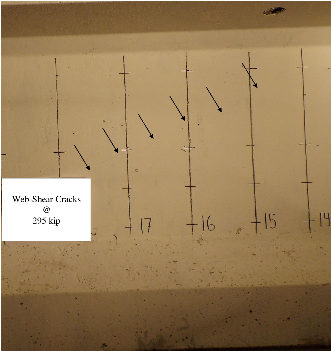
Figure 3-57: Initial web-shear cracks in 45M_8W with 295 kips applied.
