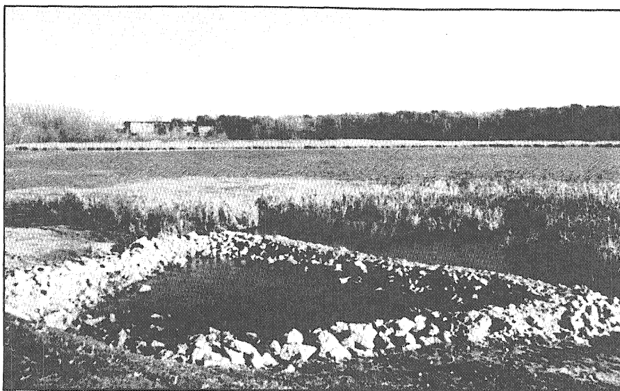
A diversion outlet running into a sedimentation basin adjacent to Little Lake Josephine.
