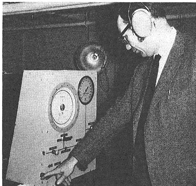
Above: Dr. Plunkett fires a gas gun. He wears ear muffs as a precaution against the sound waves resulting from the projectile hitting the plate.
