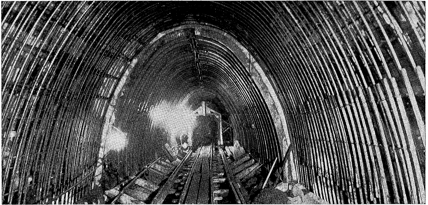
Reinforcing steel in a 13 foot-3 inch semi-elliptical tunnel section
