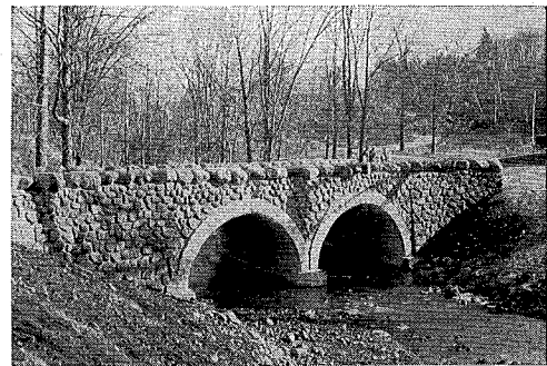
Armco Multi Plate Replacing Wooden Bridge
