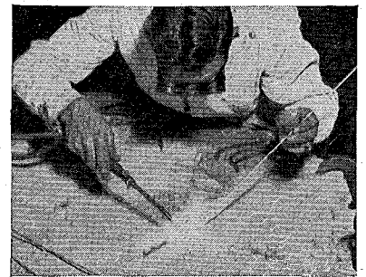
WELDING ALUMINUM—an architectural plaque, modern in design, is repaired by a modern method.
