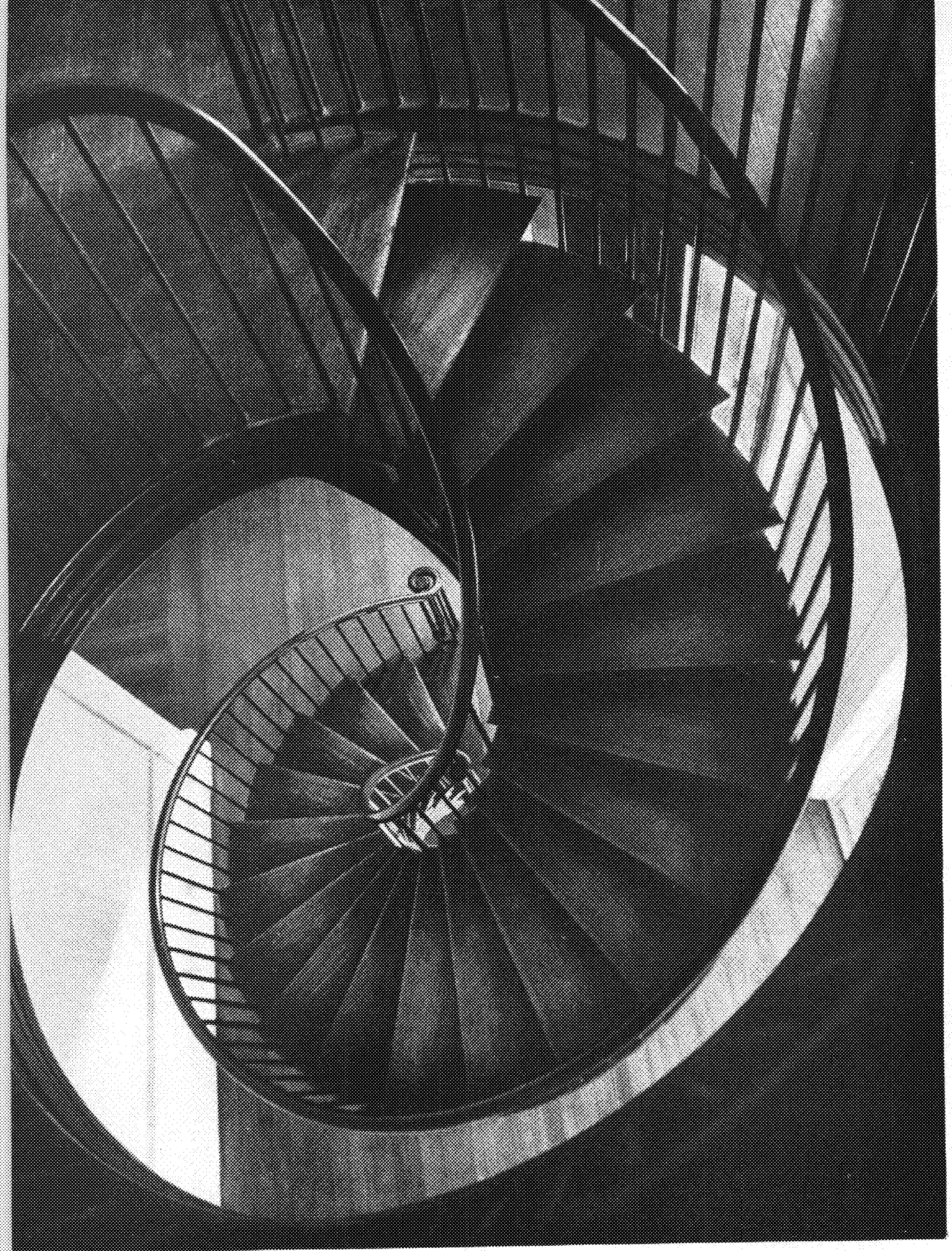
A Circular Staircase
