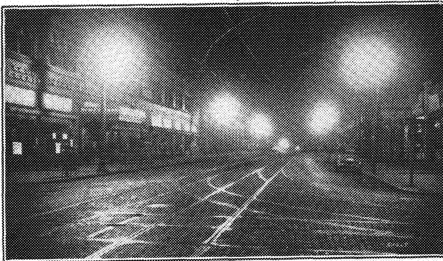
Night Turned Into Day: A Bit of First Avenue North Lighted by 1000 cp. Novalux Units Mounted at a Height of 22 feet.
