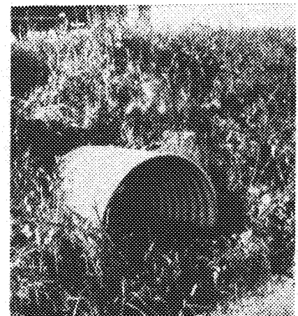
Figure 5. Metal Culvert Used 16 Years
