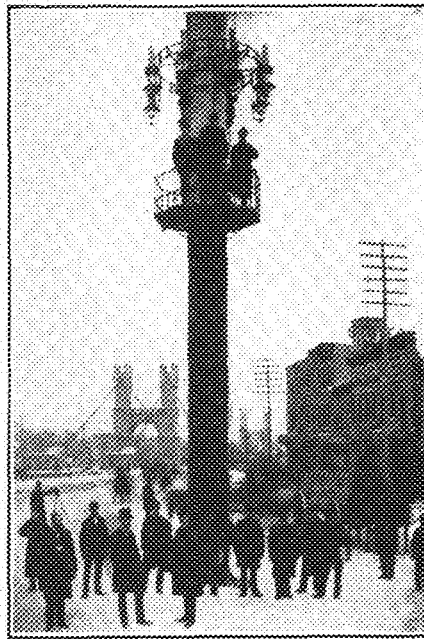
Eight Arcs on a Single Steel Tower Minneapolis' Street Lighting in 1888.
