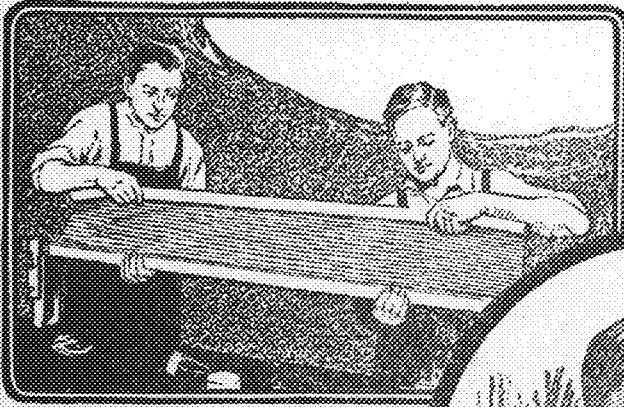
Winding high voltage insulation, 1894— 2,200 Volts
