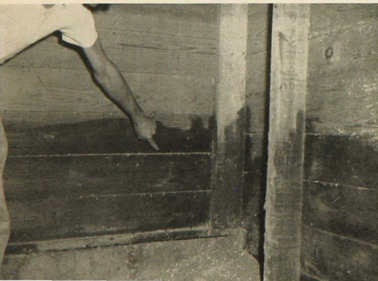
Fig. 3. A corner of a wooden bin showing the accumulation of grain in the cracks between the wallboards and on the floor.
