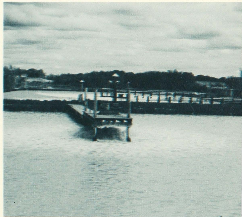
A two-stage disposal system includes chemical treatment equipment (top right) and a wastewater aerator (foreground).
