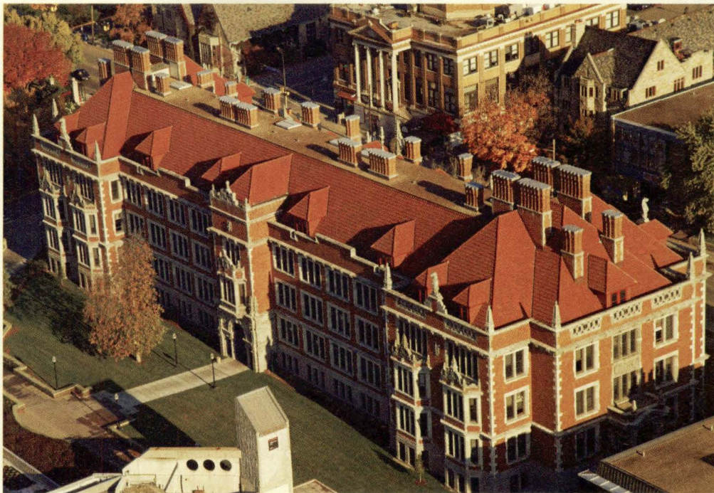
Folwell Hall was renovated inside and out. This aerial photograph was taken in October 2008, after the building's roof was repaired.
