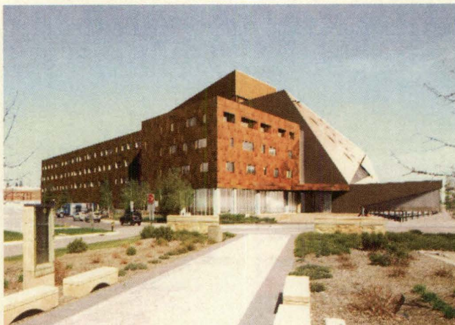
The four-story expansion to the southwest corner of the McNamara Alumni Center will add meeting and office space.
