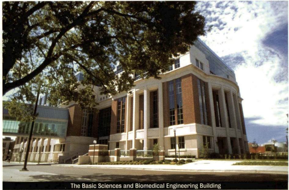
The Basic Sciences and Biomedical Engineering Building
