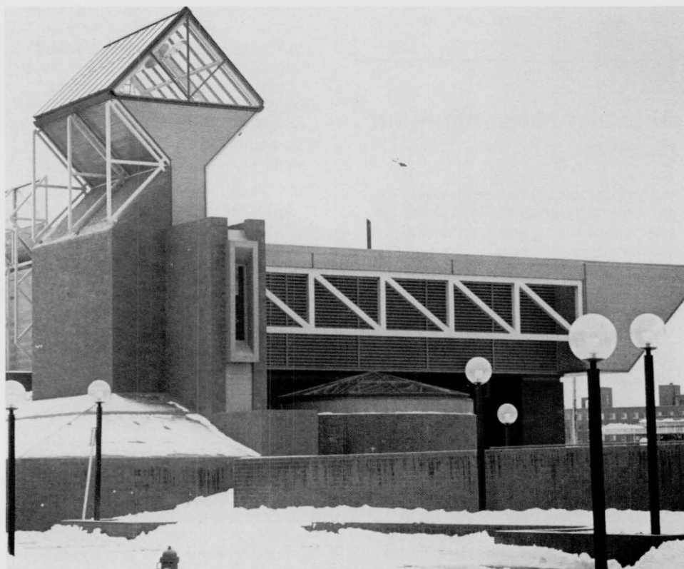
A new building for Civil and Mineral Engineering. 95 percent below ground, but far from invisible.
