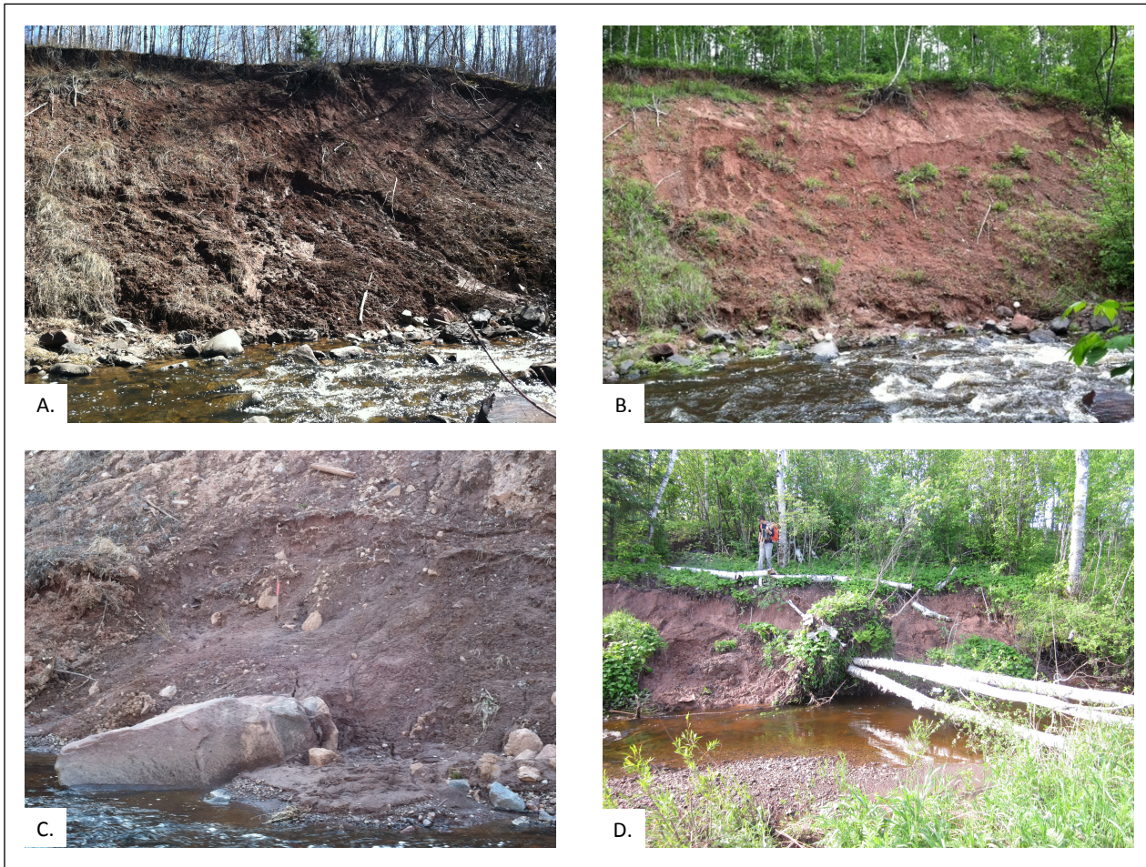
Figure 7.1: Slumps in study bluffs observed from April to May 2012. (A) Site B9 (lower main Amity); slump observed in early April. (B) Site B9; slumping continues up face of bluff following heavy precipitation May 23 to 28; significant undercutting along bluff toe. (C) Site B7 (lower Lester); slump observed in early April. (D) Site B12 (lower East Branch Amity); slump following heavy precipitation in late May
