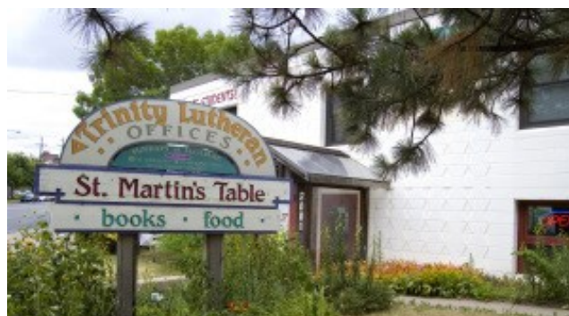
Trinity Lutheran building on Riverside Ave
