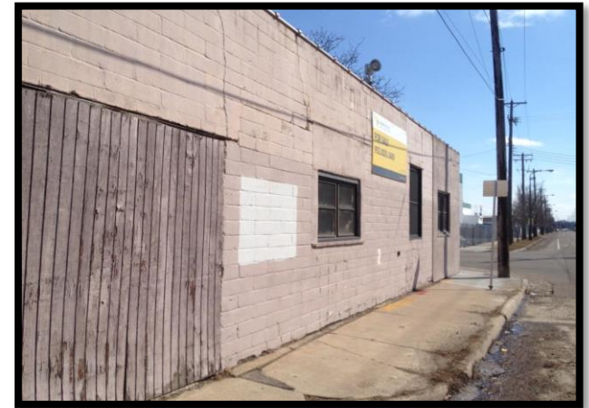
Figure 11 Example of Poor Curb Appeal
