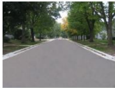
Before Permeable Pavement
