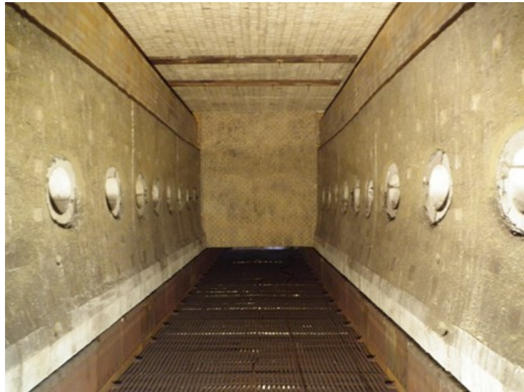
Figure 21: Furnace No. 12 Northshore Mining - Silver Bay, MN – 2012 - Furnace Reline
