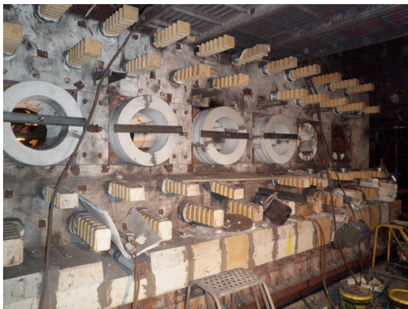
Figure 11: Furnace No. 12 Northshore Mining - Silver Bay, MN - 2013
