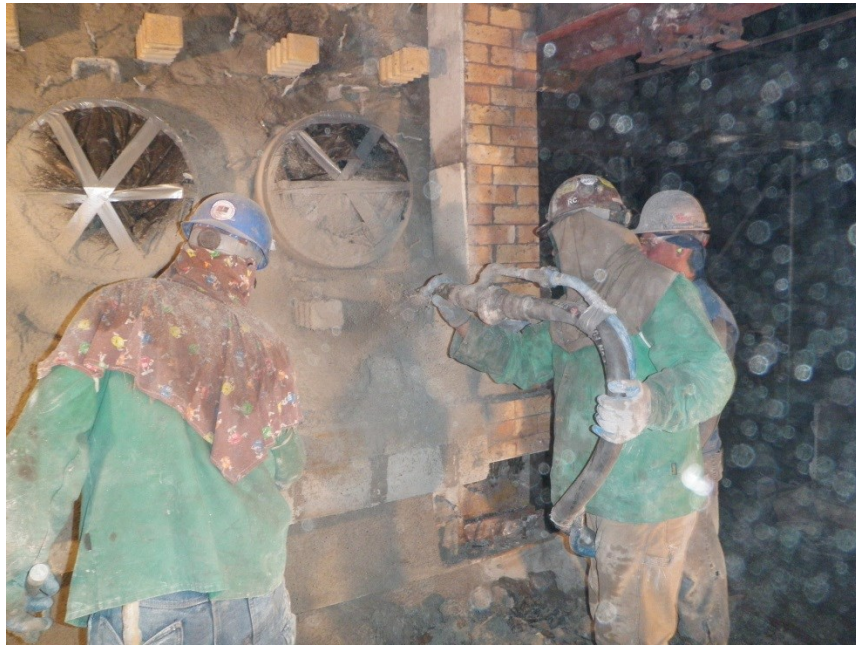
Figure 7: Furnace No. 12 Northshore Mining - Silver Bay, MN - 2013
