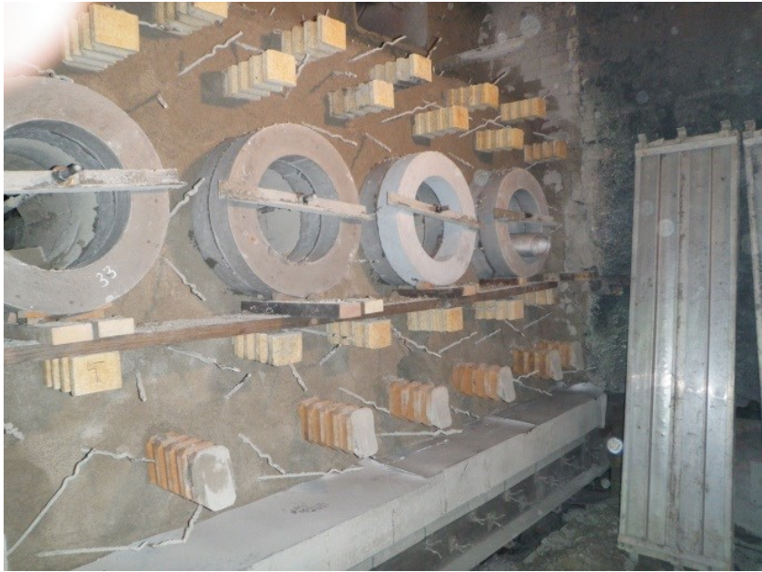
Figure 18: Furnace No. 6 Northshore Mining - Silver Bay, MN - 2011
