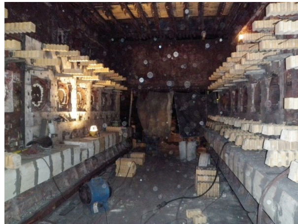
Figure 20: Furnace 12 Remote Demolition and Relining
