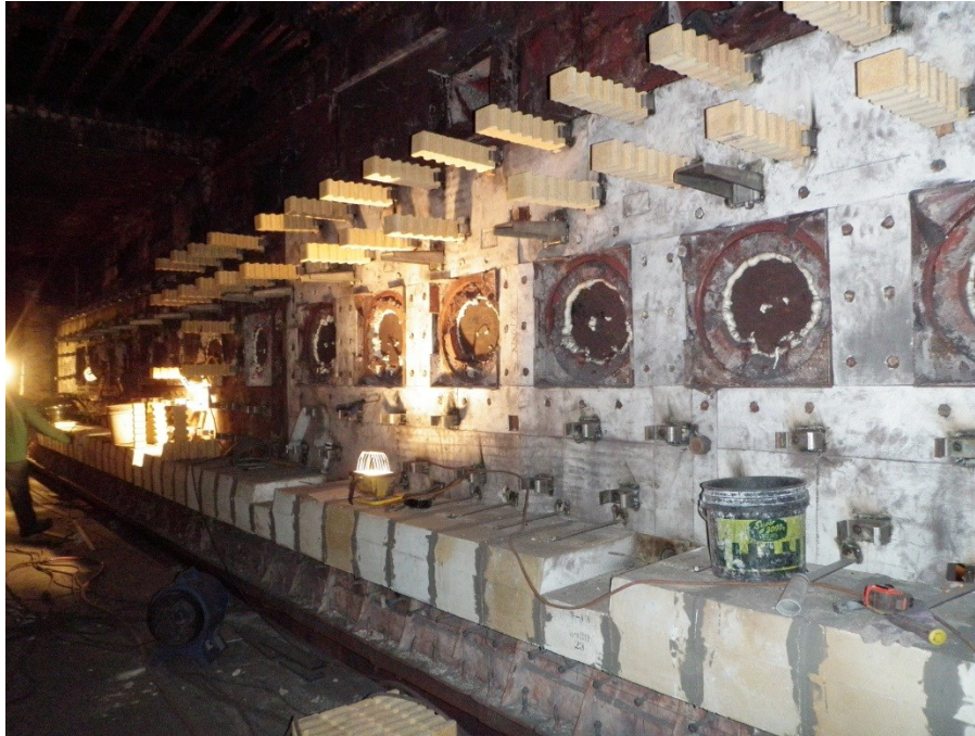
Figure 6: Furnace No. 12 Northshore Mining - Silver Bay, MN - 2013
