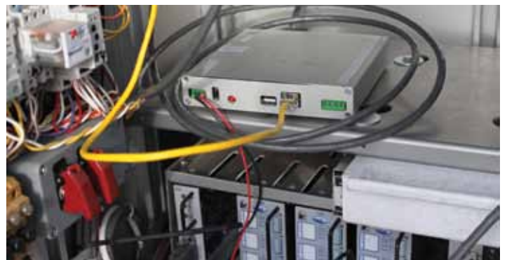
The enhanced SMART Signal system connects quickly to traffic signal controller cabinets with just a power source and an Ethernet connection.
