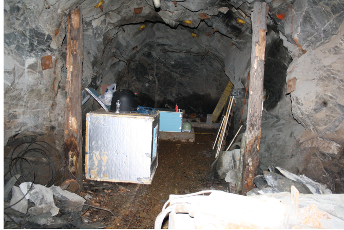
Figure 4.5: Above photo, taken during the construction of 4100ft-D station, shows the two hut setup used for isolating seismometers and data acquisition systems.
