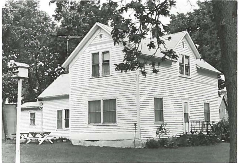
Fig. 20. Mads and Karen Bollesen house, exterior; built c. 1892.
