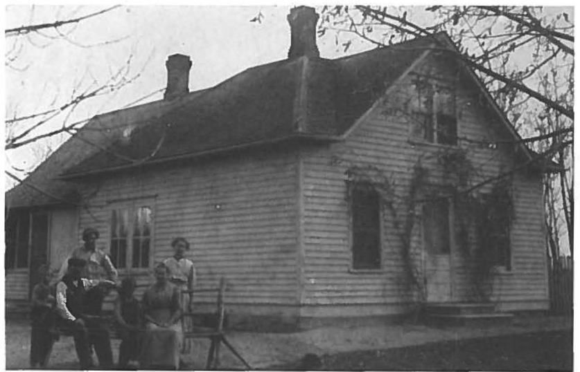
Fig. 62. Mathias and Karen Andersen house, exterior; built c. 1903.
