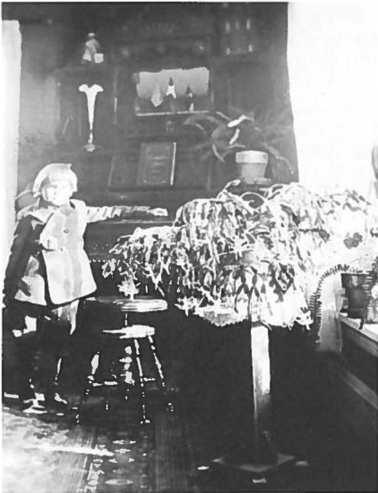
Fig. 80. Chris and Mette Utoft house, interior; living room.
