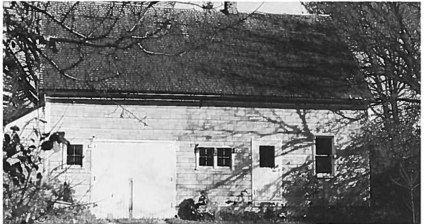
Fig. 64. Christian Howe house, exterior; built c. 1900.
