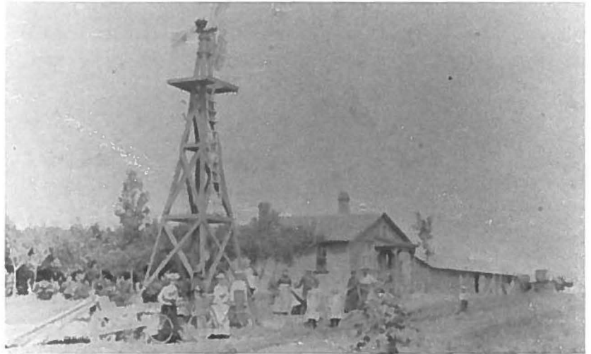
Fig. 69. Hans Peter Christian and Sine Hansen house, exterior; built c. 1889.
