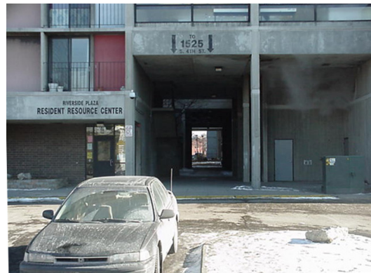
18 Right of Way Corridor Looking from Site
