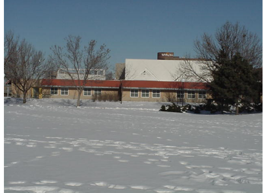
Brian Coyle Center Looking North 11
