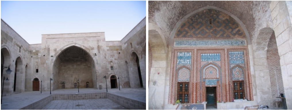
Figure 4.2 Views from the main iwān (left) and tomb section (right) of the hospital during its in-progress restoration in 2011. Source: Photos by the author.
