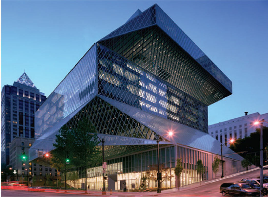
Figure 5: Exterior Photo of Seattle Central Library.
