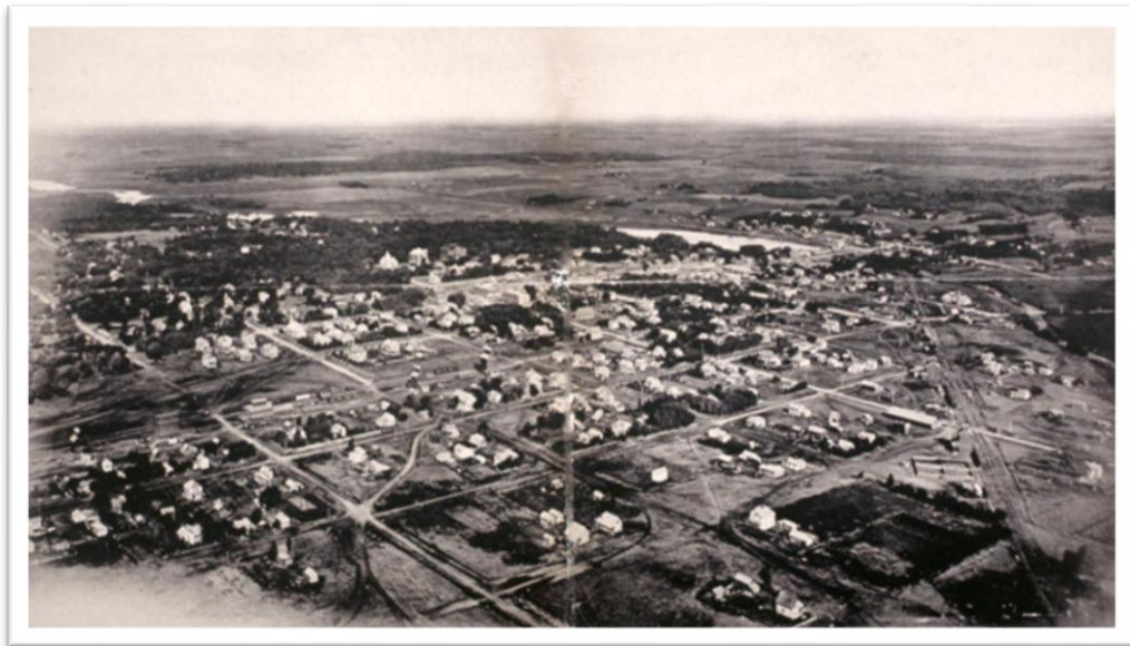
Figure 5. Historic panoramic view of Hutchinson from 1901 (image from LakesnWoods.com courtesy US Library of Congress, original photo from Minneapolis Tribune Company).
