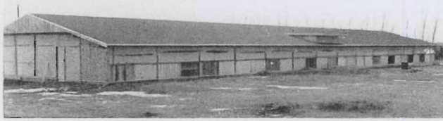
Fig. 4. Pole frame turkey shelter building, 54 x 196 feet, insulated and ventilated and built largely from Minnesota pine.
