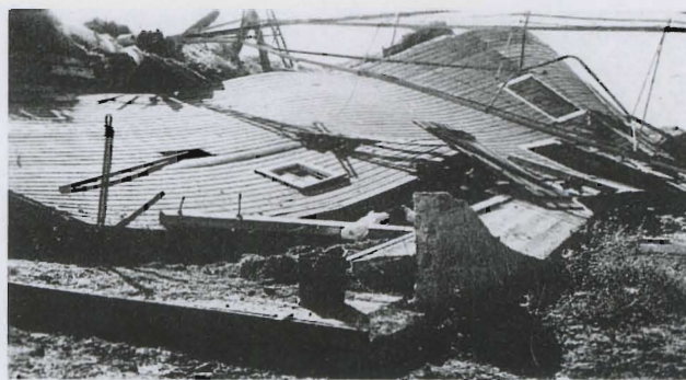
Fig. 1. A shallow foundation wall without footings or reinforcement.
