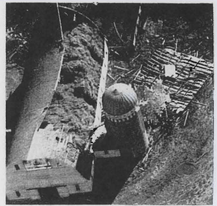
Fig. 6. This is a typical roof failure due to wind action. The wind direction was from left to right.
