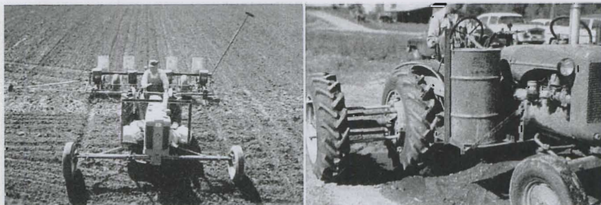
Fig. 3. Four-row wheel-track modification devised by Rollin Dennistoun at the Rosemount Experiment Station. The one at left was used in 1957, the one at right in 1958.
