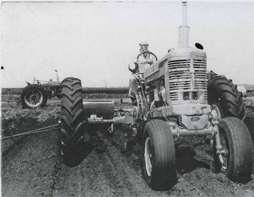
Fig. 4. Four-row wheel-track modification, courtesy Schwartz Manufacturing Co., Lester Prairie.
