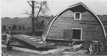
Fig. 5. This failure resulted from a lack of knee and wall braces.
