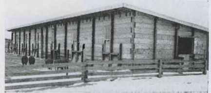
Fig. 6. A pole frame, uninsulated hog shelter built with treated poles on outside of 2-inch plank walls.
