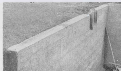
Fig. 2. A foundation wall without anchor bolts.
