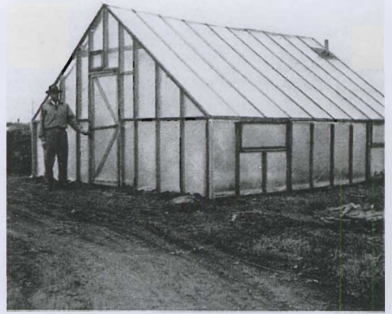
TEST STRUCTURE built in the fall of 1955. Several different thicknesses and types of plastic film have since been tested.
