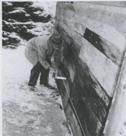
Fig. 3. Walls bulged when posts for this silo were spaced 6 feet apart. A 4-foot spacing of posts on the other test silo resulted in very little bulging.
