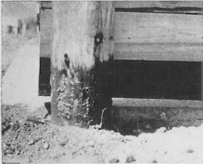
Fig. 2. A 1-inch gap between cement floor and walls provided the test silos with excellent lateral drainage.
