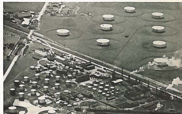
Fig. 6. Air view of a cooperatively-owned refinery and petroleum tank farm.
