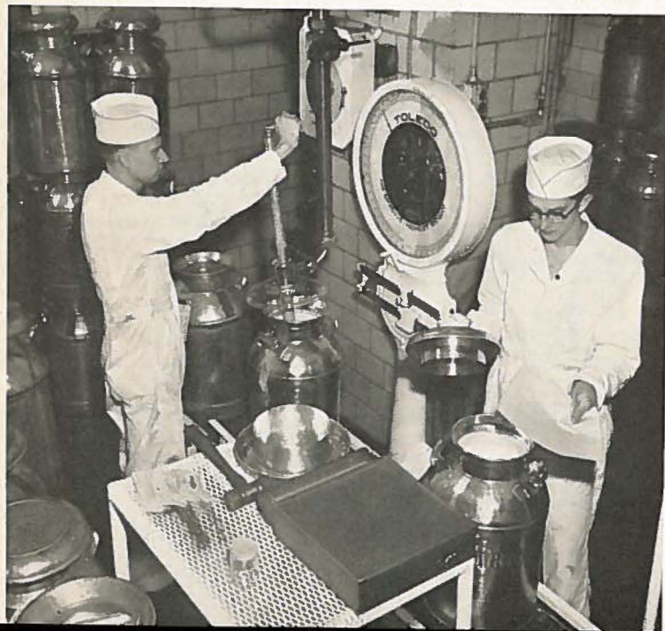
FIG. 5. Filling cans with 40 per cent cream for out-of-state shipment. Fluid milk, condensed milk, and ice cream mix also are shipped by many plants.
