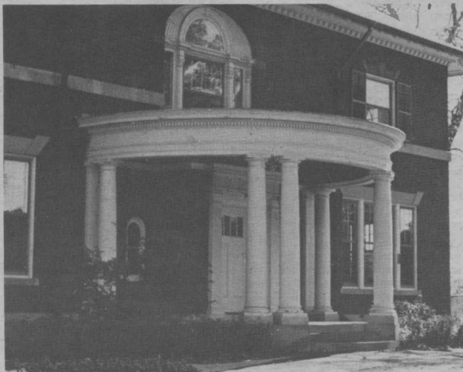
An attached entryway, a vestibule-like space that prepares one for entering the sanctum of the house.
