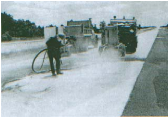
Figure 7: An example of a sandblasting surface preparation (Smutzer 1993)
