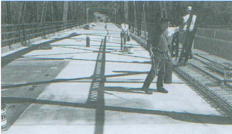
Figure 14: An example of a deck sealant applied using hand sprayers (Whiting)
