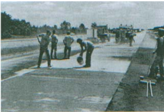
Figure 15: An example of a flood coat (Smutzer 1993)
