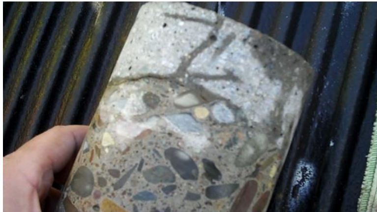
Figure 5-23. Core showing debonding of the partial depth repair.
