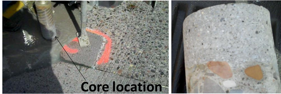
Figure 5-19. Core location (left) and result showing properly bonded partial depth repair.
