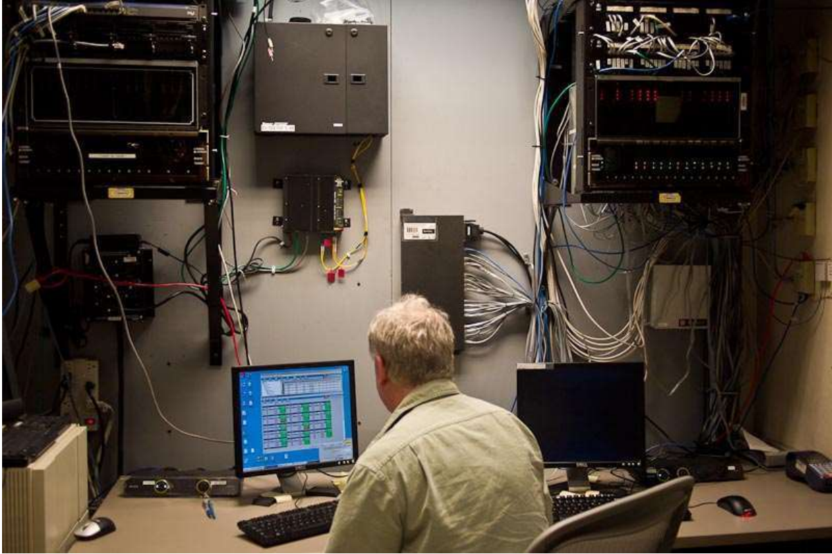
Monitoring Parking Ramps, Parking and Transportation Building
