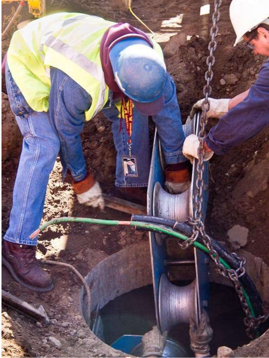
Pulling Wire in Preparation for Light Rail Construction
