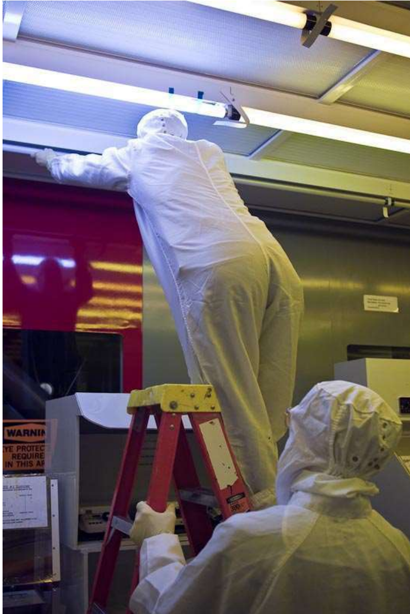
LED Installation, Keller Hall
