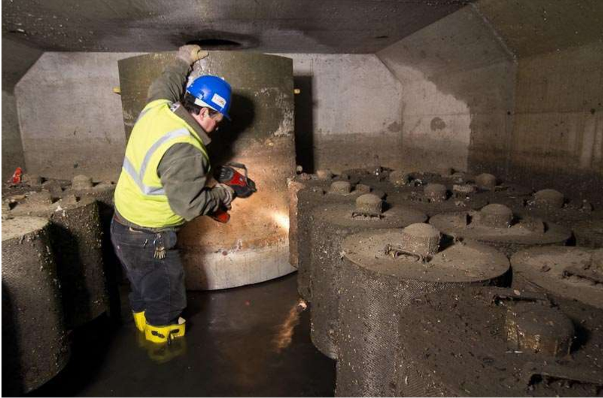
Checking Rainwater Runoff Filters at TCF Stadium
