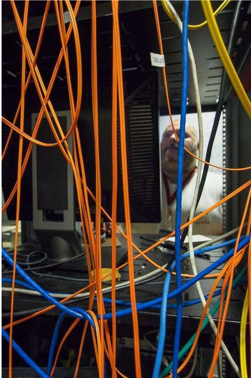
Building Systems Automation Center, Facilities Management, Donhowe Building
