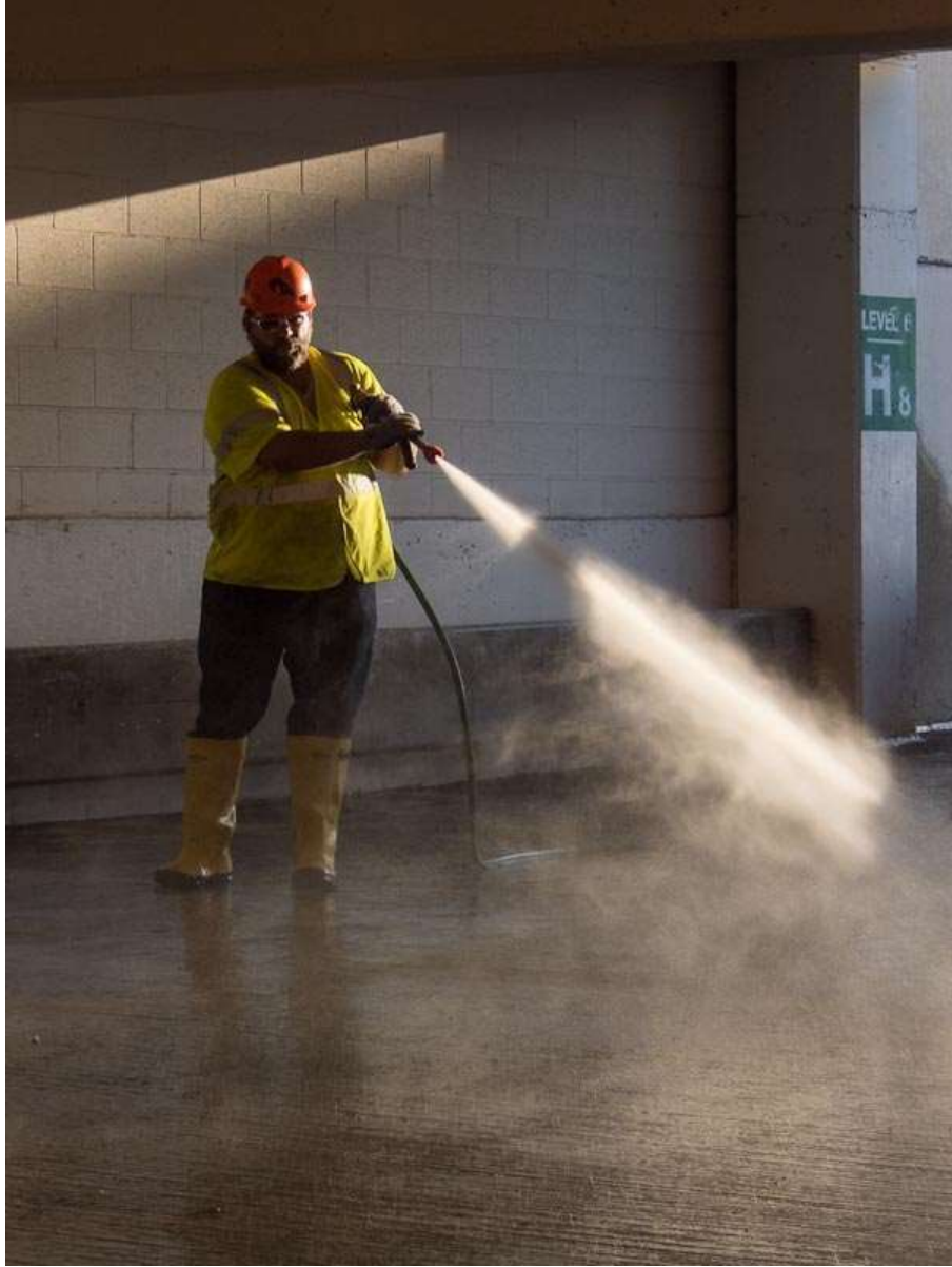
Power Washing the Washington Avenue Parking Ramp
