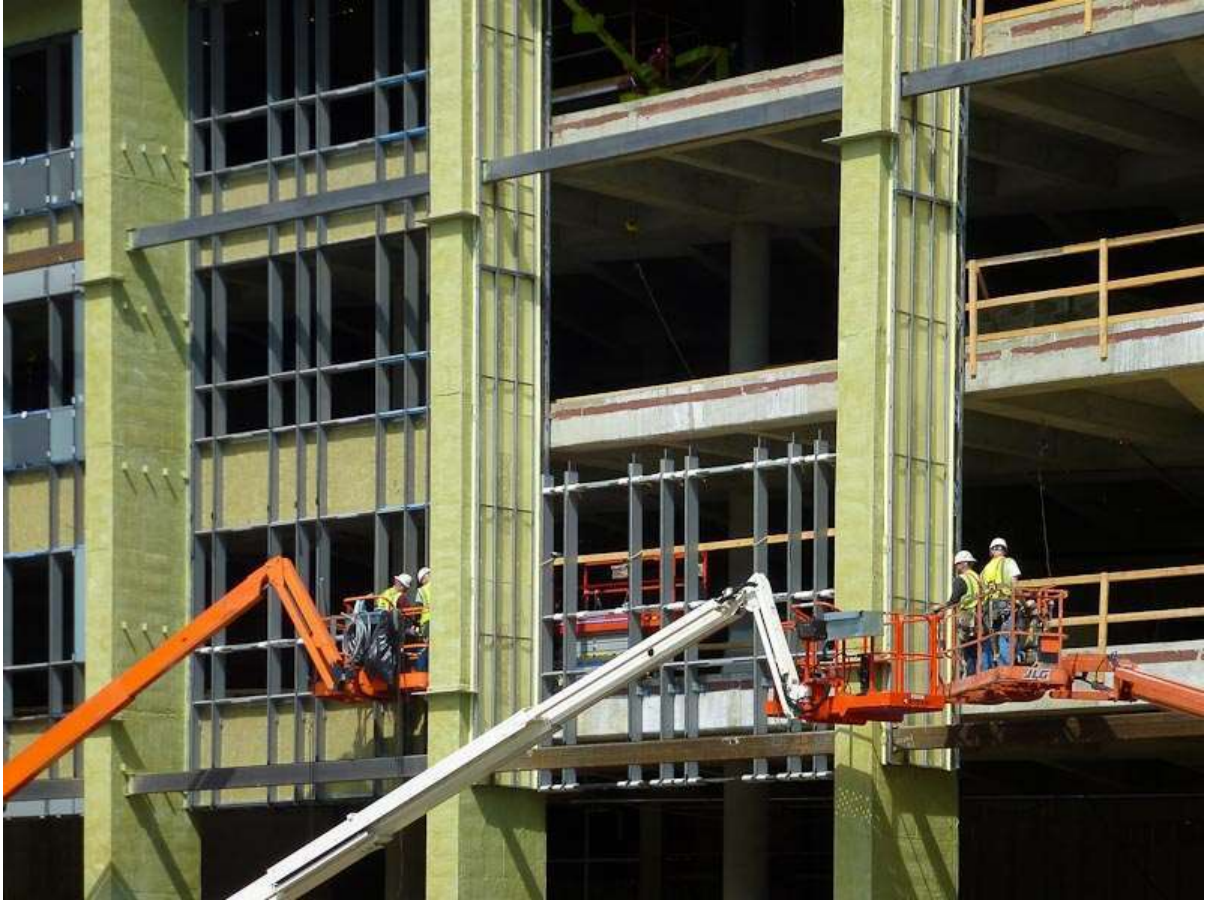
Recreation and Wellness Center Construction
