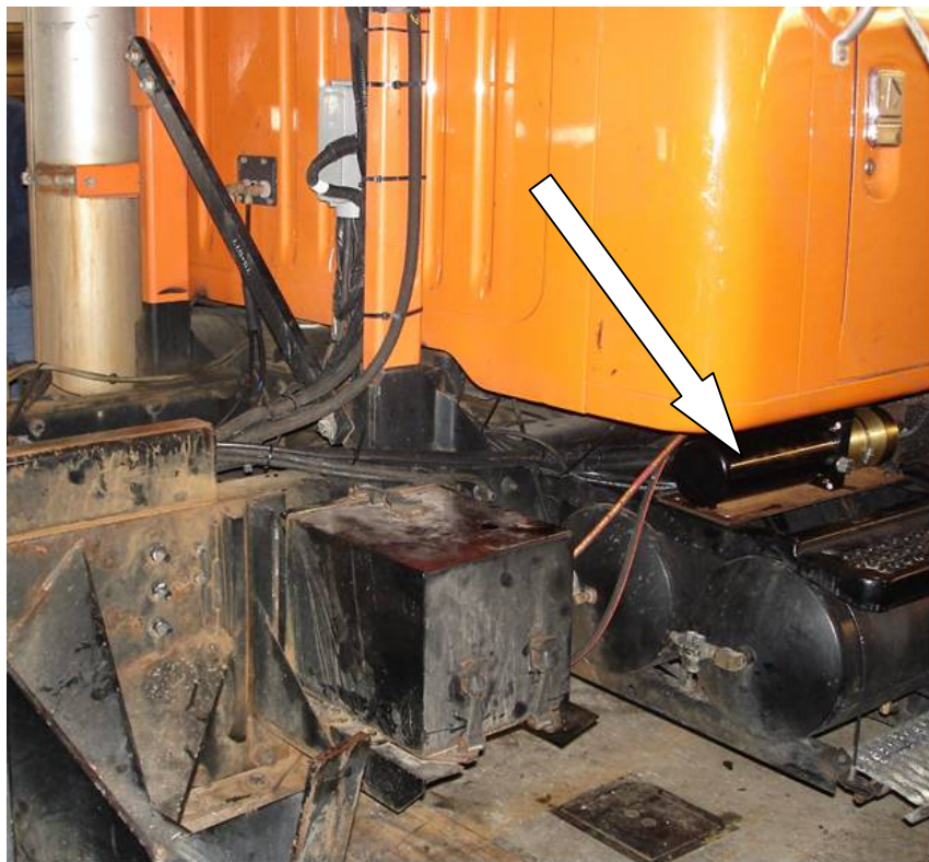
Figure 6.15: Hydraulic Power Unit Mounting
