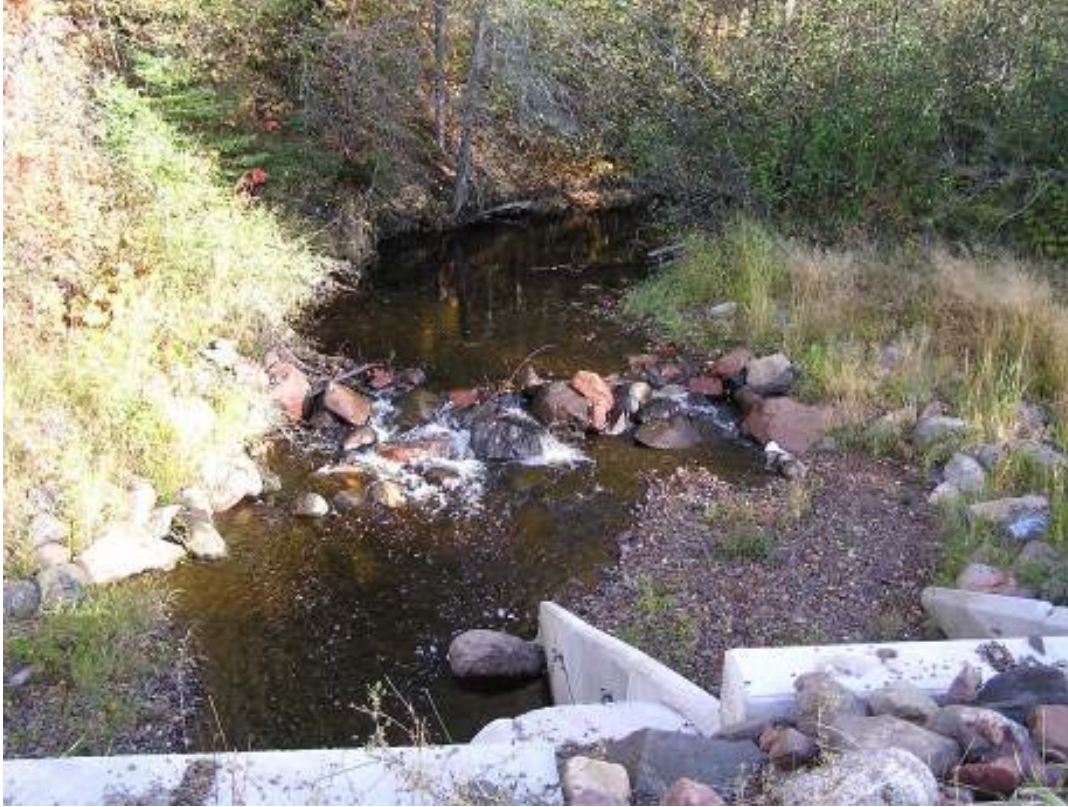
Figure 5.2. Photograph of rock placed in the channel immediately above the culvert to protect against head cut development.
