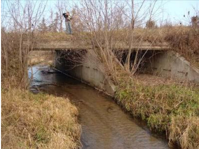
Figure 5.3. Photograph showing a highly mobile sand bed at Gorman Creek. Note the side culvert filled in with sediment (Goodhue County).
