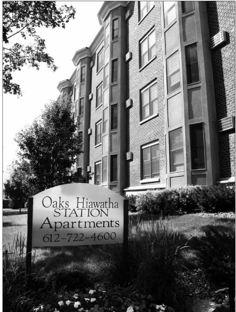
Housing along the Hiawatha light-rail transit line
