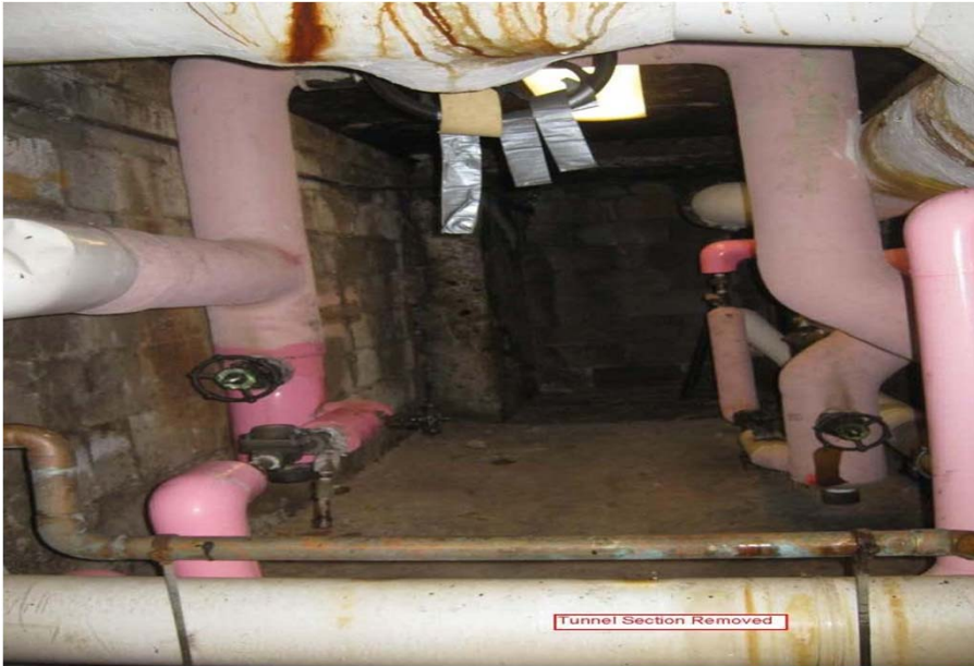
1940 Construction Steam Tunnel: Crumbling block walls under a St. Paul roadway
