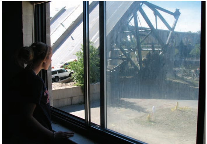
A view of the I-35W Bridge collapse from the University's Tandem Accelerator Building. OGC worked on a number of significant legal issues related to this tragic event.
