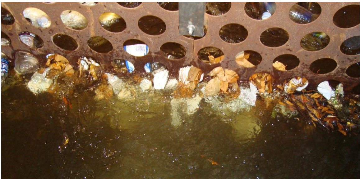
Figure 2-8: Debris stuck in the SAFL Baffle during Test 2. The view is from near the outlet pipe, looking upstream.
