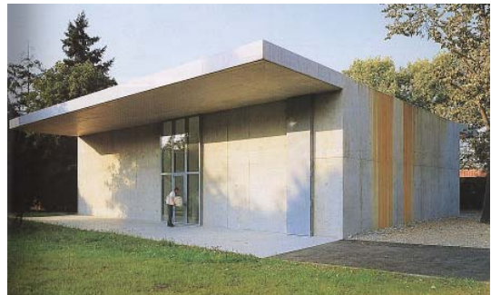
Fig. 35 EXTERIOR VIEW OF THE STUDIO.
