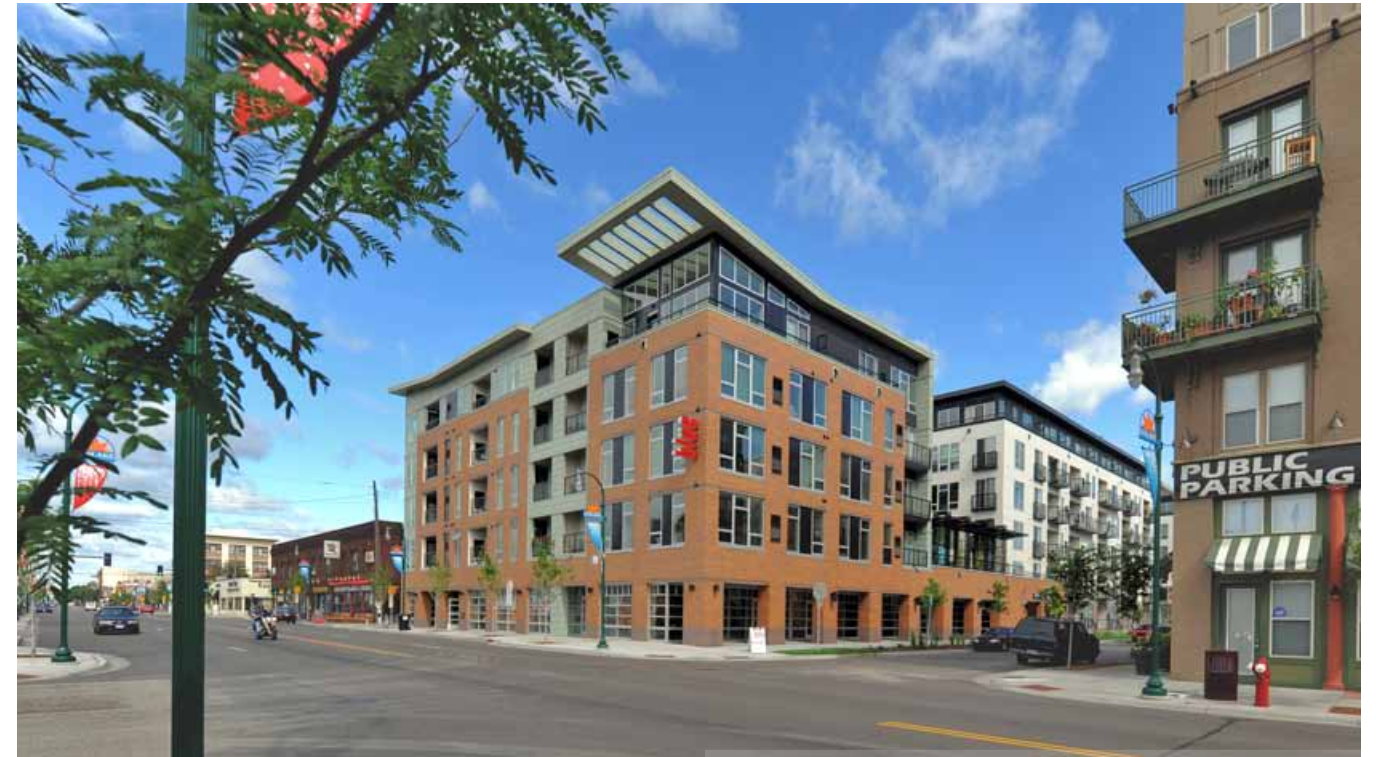
(ABOVE) Looking northwest across the intersection of Lake St and Aldrich Ave in the Lyn-Lake area, which is one in a string of nodes along Lake St. The awnings along the roofline facing south are to minimize solar heat gain in the summer, but allow in low-angle sun in the winter. (Image used with permission from the BKV Group, www.bkvgroup.com )
