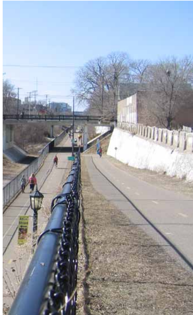
(ABOVE) This photo is typical of the ramps leading from street grade down to the Greenway (approx. 30' in elevation change, depending on the location). This particular photo was taken at street grade, Nicollet Ave just north of the Kmart building, looking west toward Blaisdell Ave.
