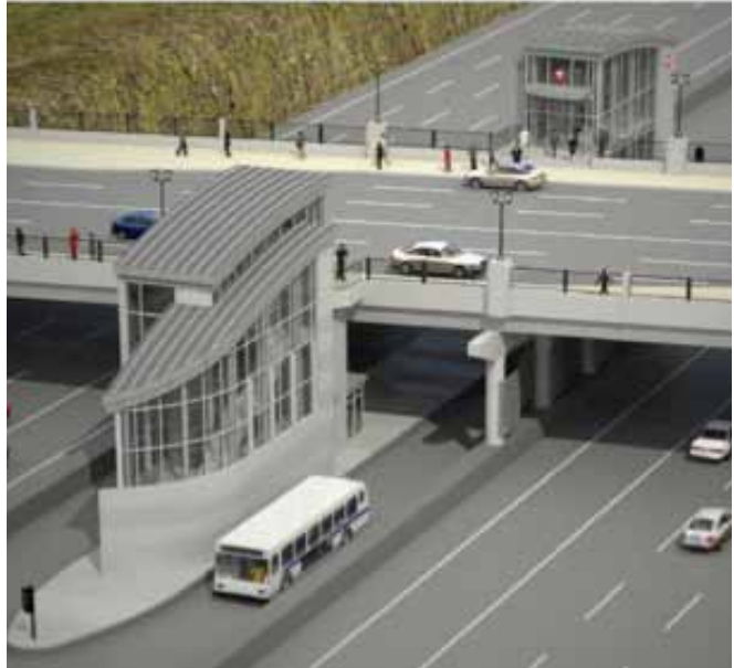
(ABOVE) The Franklin Ave LRT station is used as an example, because it spans the roadway beneath, connects to other transit services (note the Metro bus), and provides room for services under the track alignment. Given the potential streetcar stop above the Greenway at Nicollet (see the previous page), there could potentially be amenity space for bike parking, lockers, or showers in the station on the Greenway.
