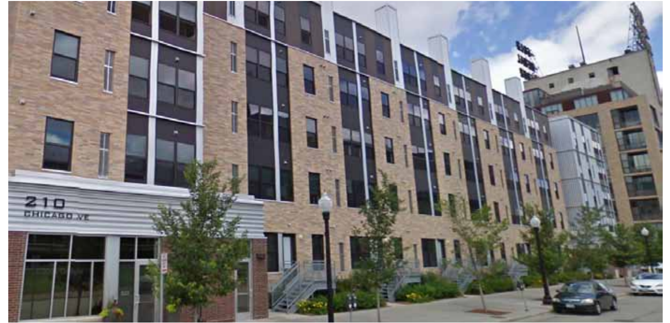
(ABOVE) The eastern facade of the St. Anthony Mills Apartments is a five-story residential facade, with individual unit entrances. The south facade, facing Washington Ave, is mixed-use with the bottom story housing 4 local businesses including both retail and office uses.
