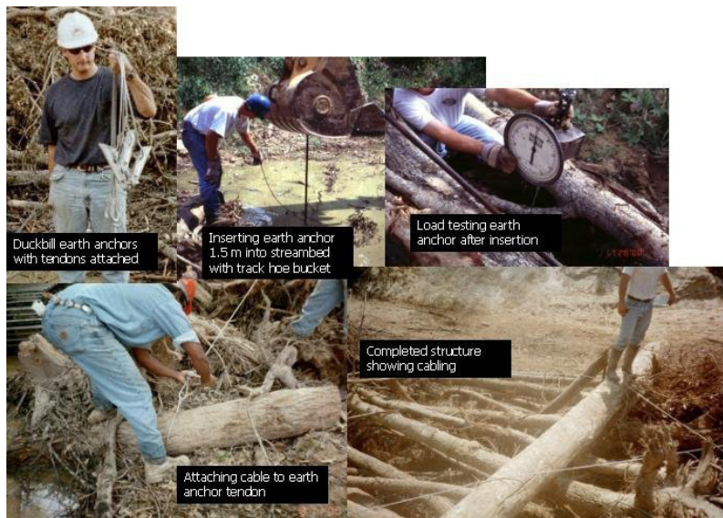
Large woody debris structure in the making.
